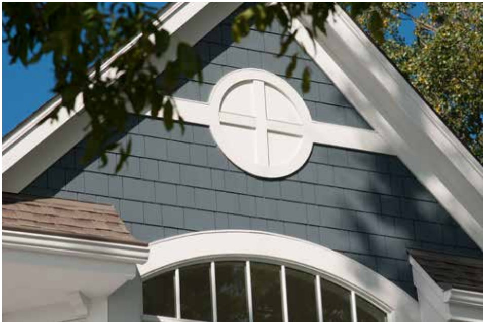
HardieShingle® Siding Straight Edge Panel Evening Blue HardieTrim® Boards Smooth Arctic White
